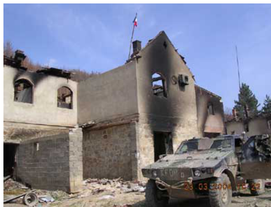
Devic Monastery ruins (a 15 th century monastery) looted and vandalized repeatedly during and after the war
